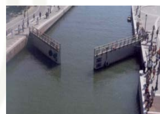
The «Porte Vinciane»: a sea gate to protect the harbour entrance
